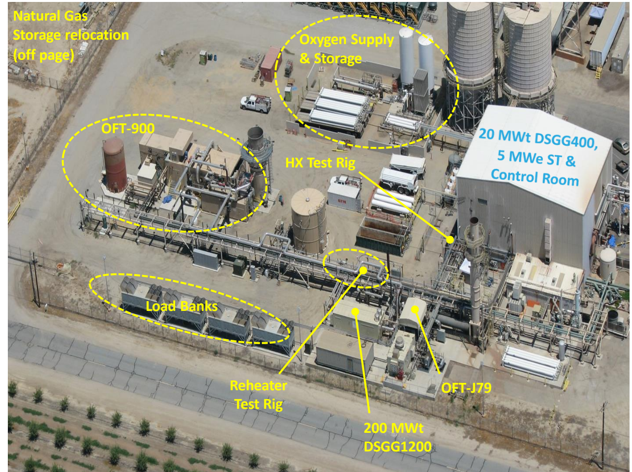
Aerial image of the Kimberlina Power Plant (KPP) Test Facilities, Bakersfield, CA; Not Shown: CO 2 supply system
