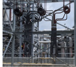
Final Header Assembly
