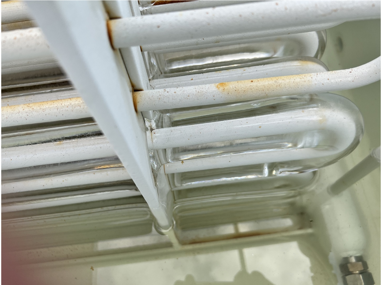
Figure 6: Ice formation on the IOC tubes during trail run of the installed system.
