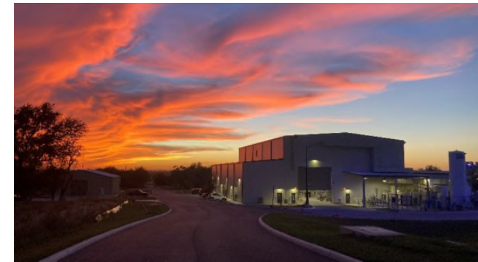
STEP Facility in San Antonio, TX
