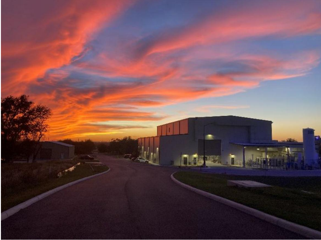
Figure 1 STEP FACILITY IN SAN ANTONIO TX
