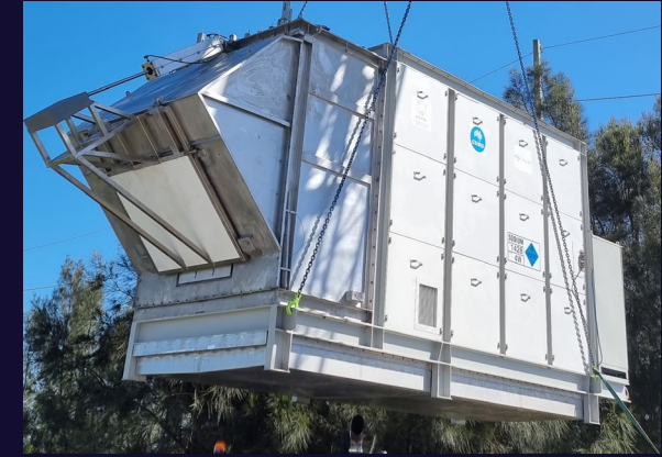
Sodium Receiver 740 °C
