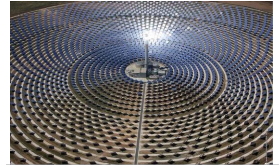
Concentrating Solar Power
