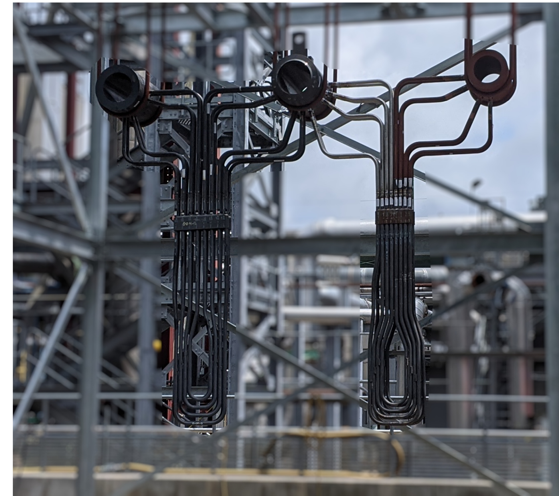
Final Header Assembly
