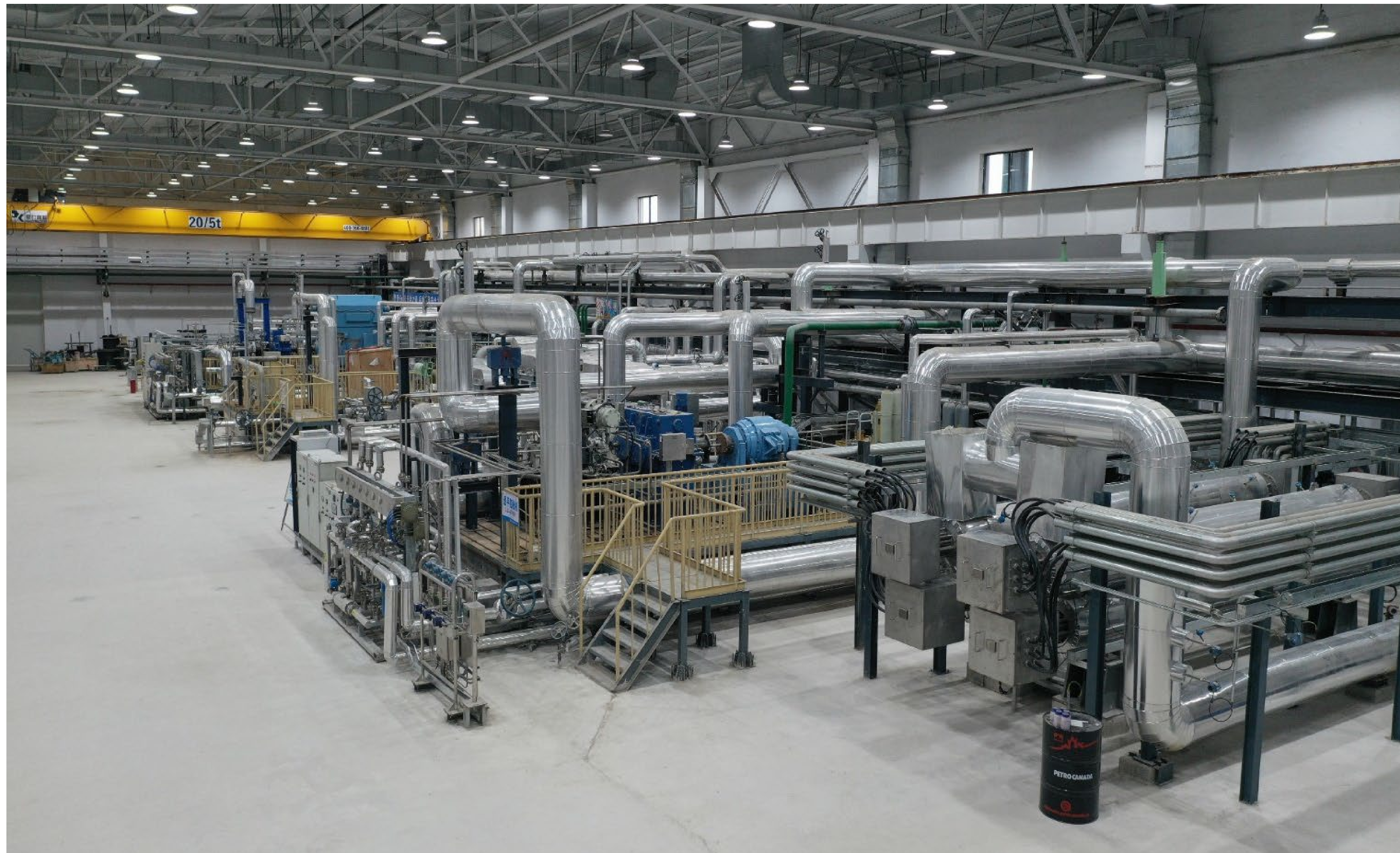
View of test bench construction in the plant(Shanghai)
