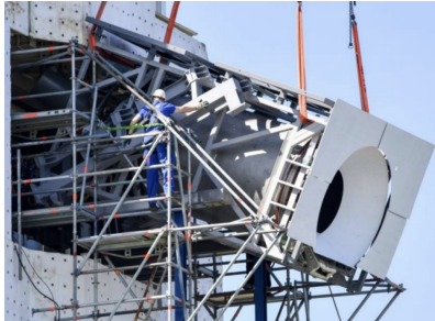
Figure 6: Real centrifugal experimental receiver by DLR. [38]
