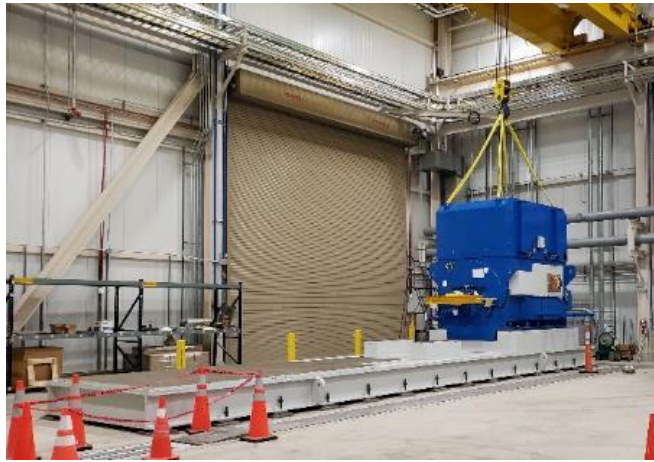
Figure 21 - Turbine Skid with Generator Installation
