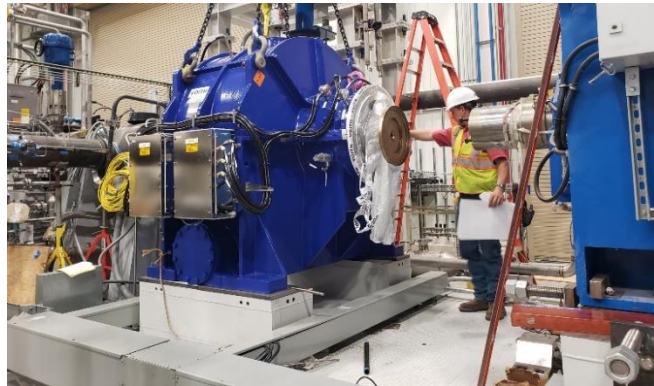
Figure 22 - Gearbox Installation on Turbine Skid
