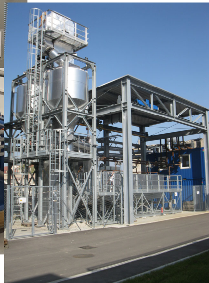
High-Temperature Reservoir (HTR)
