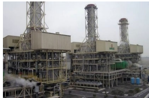
Waste Heat Recovery
