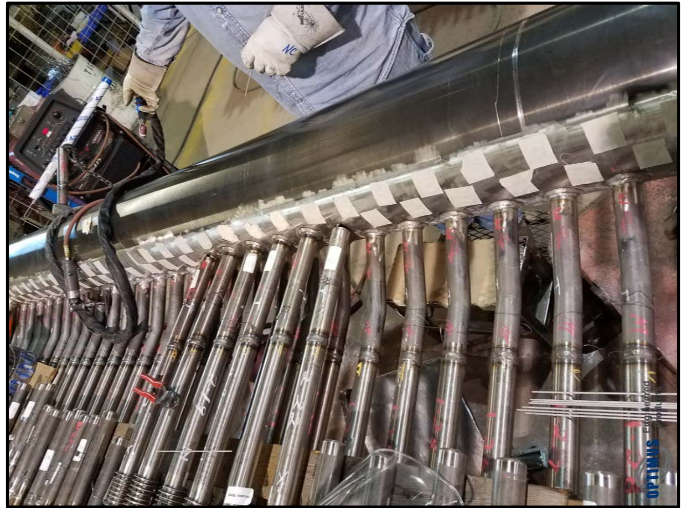
Tube-to-header welds (set-on design, 292 welds total)
