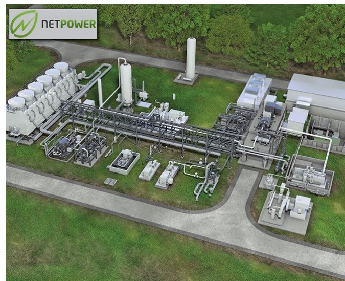
Direct fired sCO 2 plant by NET Power
