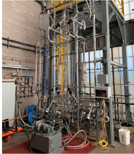
Heat Exchanger Testing
