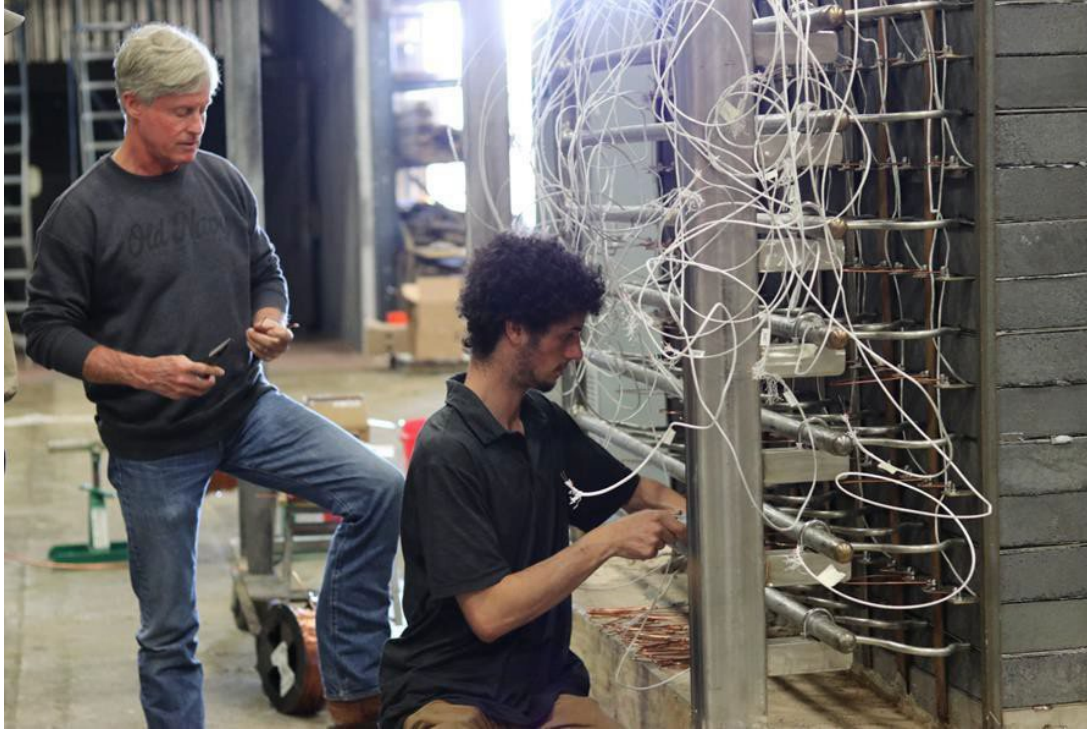
Figure 4– Assembly and Wiring of the TES Vault Internal Heaters and Instrumentation
