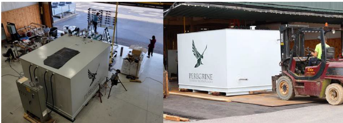
Figure 5- Delivery and Installation of the Peregrine Thermal Energy Storage Vault
