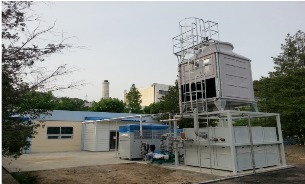
Figure 3. The picture of SCIEL building (outside)
