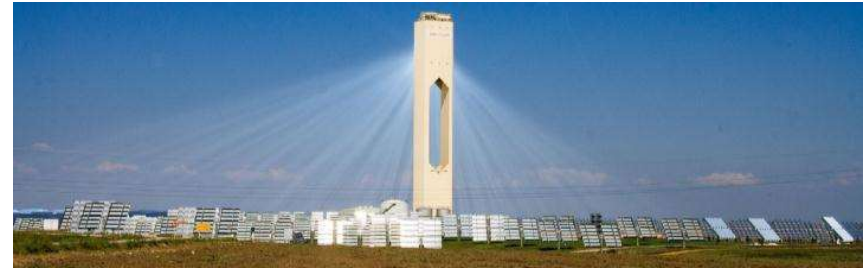
DOE Sun-Shot sCO 2 Brayton Cycle: 1MW Closed Cycle Test Facility
