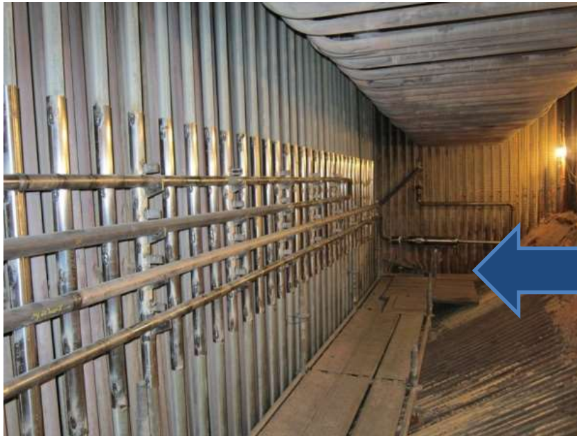
Southern Company – Plant Barry
