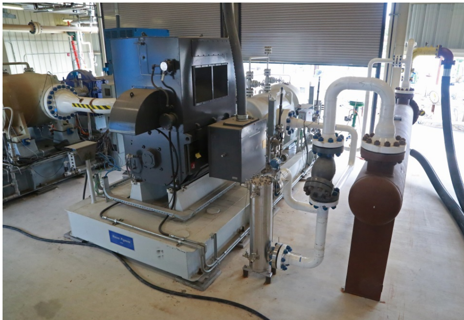
Figure 12. SunShot Piping Connecting the Pump to the Loop
