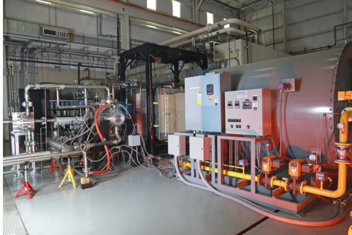
Figure 11. SunShot Piping in the High Bay Laboratory of Building 278
