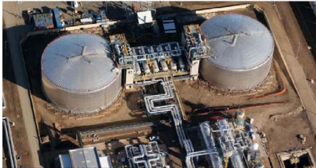
(a) 8 hours of storage for a 50 MW CSP plant using molten salt operating in Andasol 3, Spain
