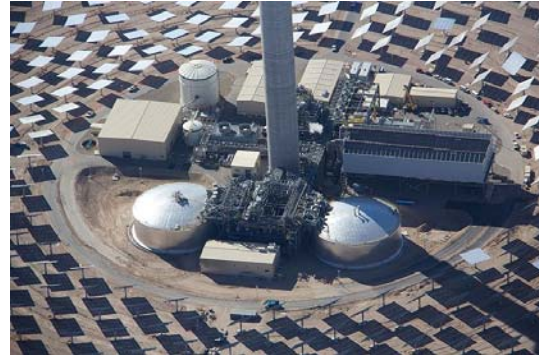
(b) 10-12 hours of molten salt storage for a 100 MW solar plant at Crescent Dunes, CA, USA
