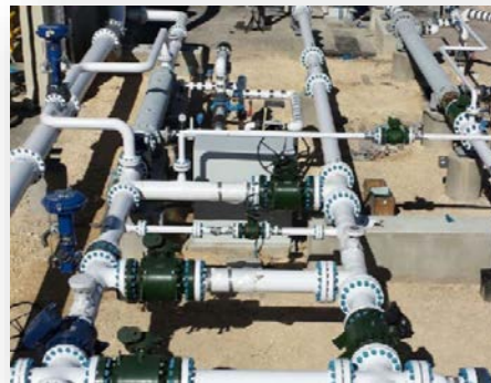
CO 2 Liquefaction Loop
