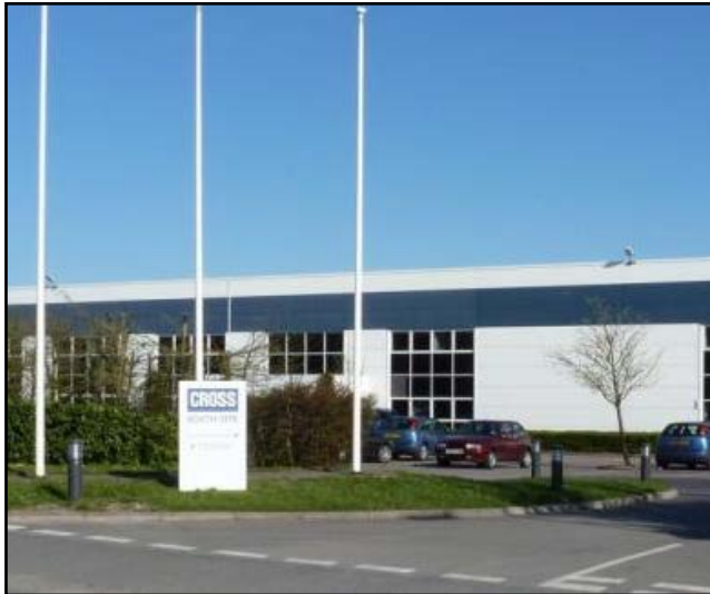
Brush Seal & Aerospace Division Devizes South Site
